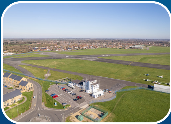
Control tower and runway improvements
