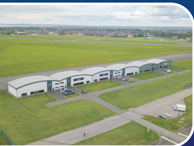
Six new hangars completed in 2018
